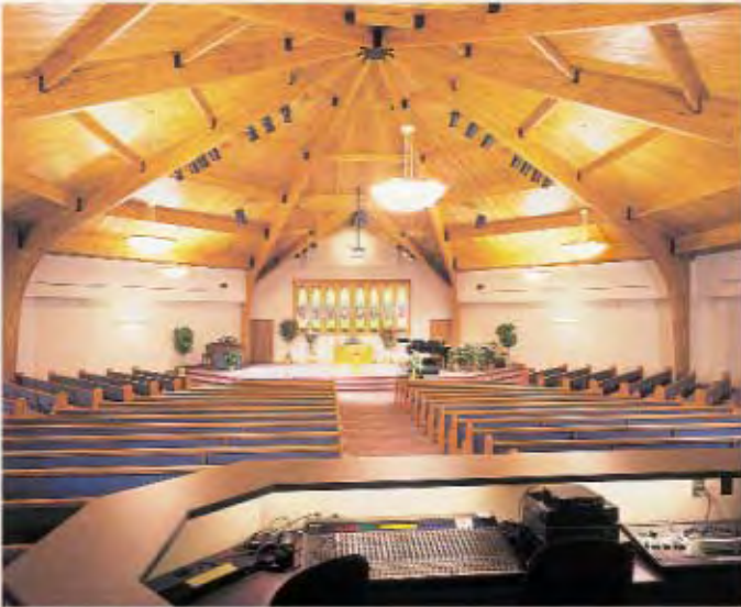
Rockbridge series pendants with optional quartz down-lighting illuminate this beautiful sanctuary in Lafayette, Indiana.
